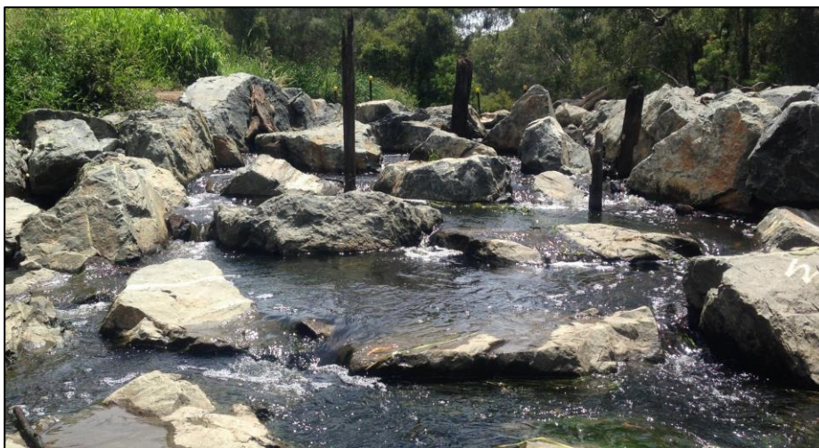
Figure 3. Facing upstream at the fishway; showing pools, ridges, and 'V'-slots (gaps between ridge rocks that fish swim through which also control the height of each pool).
