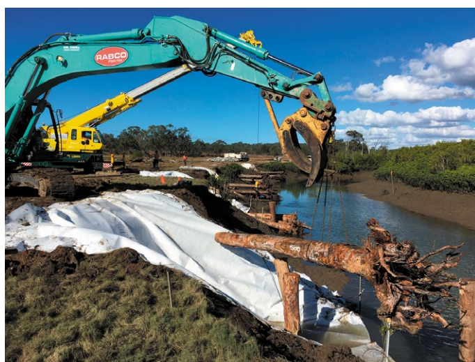
Crane & Excavator lowering logs into position - Clyde Creek
